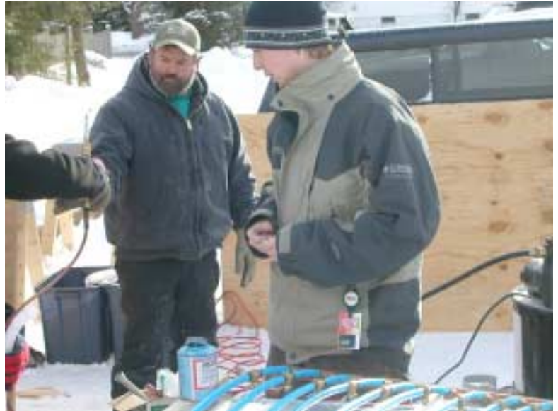
ABOVE and BELOW: Students learning and applying the basics of pipefitting with local experts.
